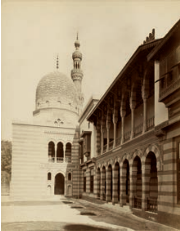
Figure 8. A building imitating the Wikala at the other side of the center of the Egyptian pavilion, Vienna 1873, see Vienna Museum online catalogue.
